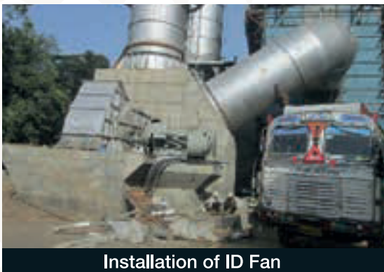
Duct Erection
